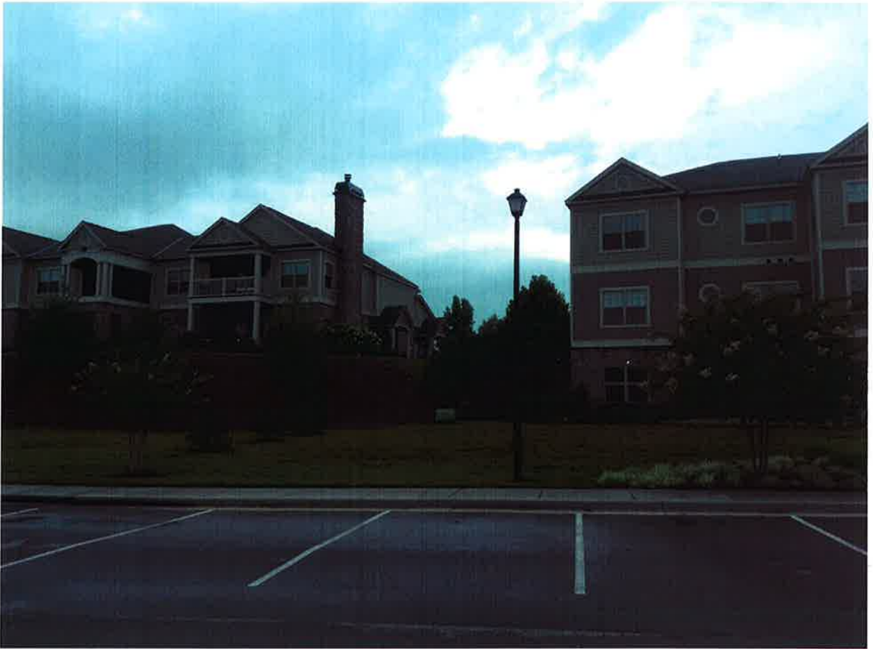
Two Story & Three Story Buildings
