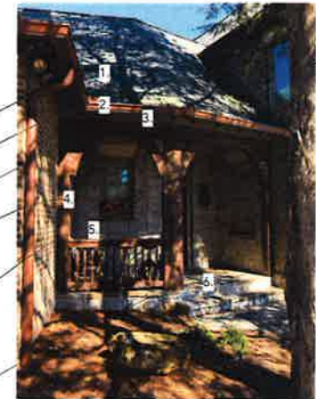
EXISTING SIDE PORCH
