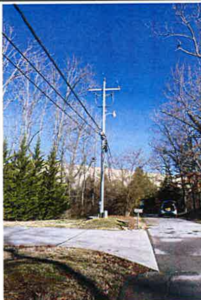
EXISTING SITE STRUCTURE
