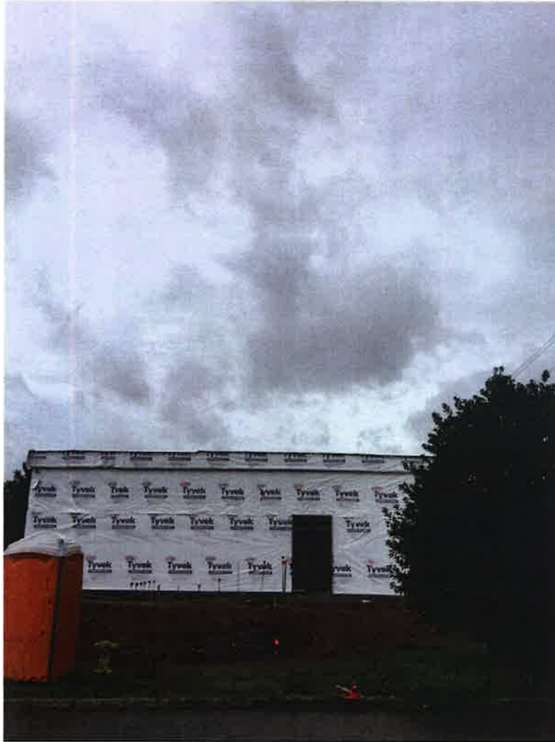
CURRENT VIEW (FROM NE LOOKING SW)
