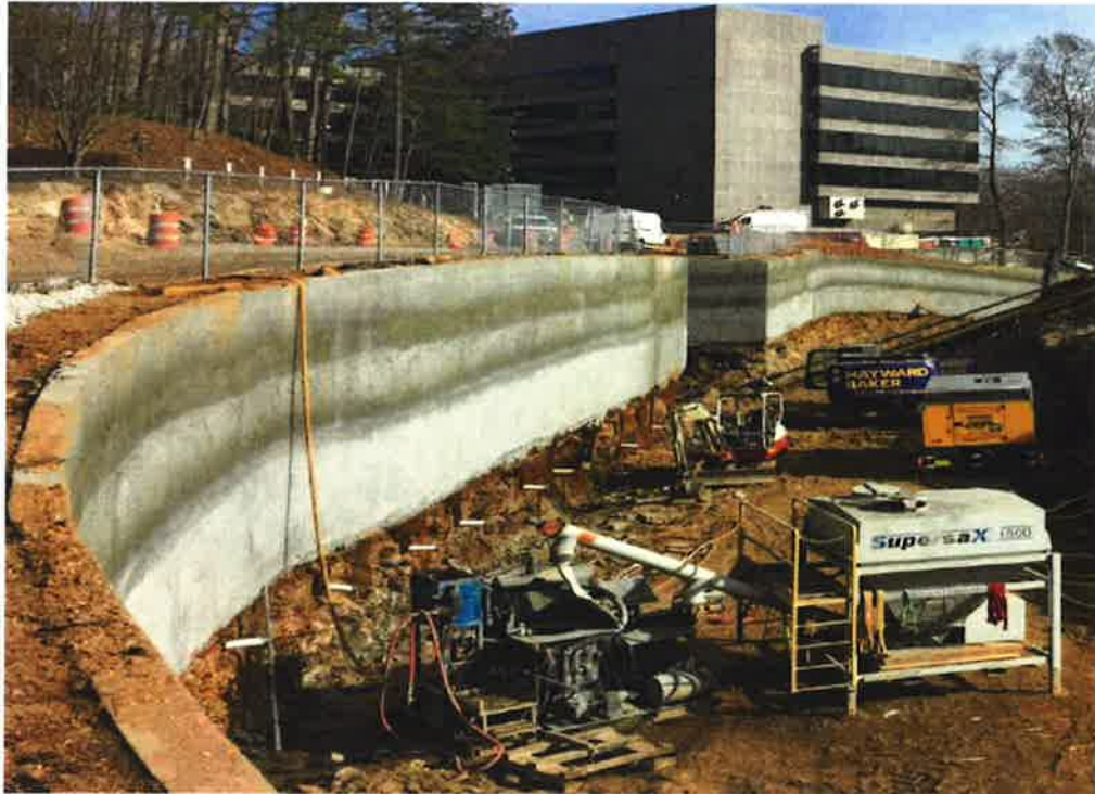
Broadstone Juniper, Atlanta, GA 2015 15,000 SF Soil Nail Wall w/ Screeded Finish and Formed Top of Wall
