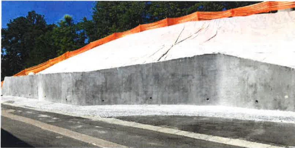
Heards Ferry Elementary School, Atlanta, GA 2014 18,000SF Soil Nail Wall w/ Rubbed Finish and Formed Top of Wall
