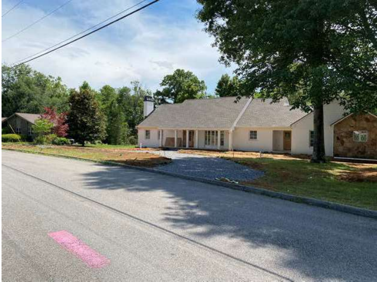
Monticello Drive right view of circular drive
