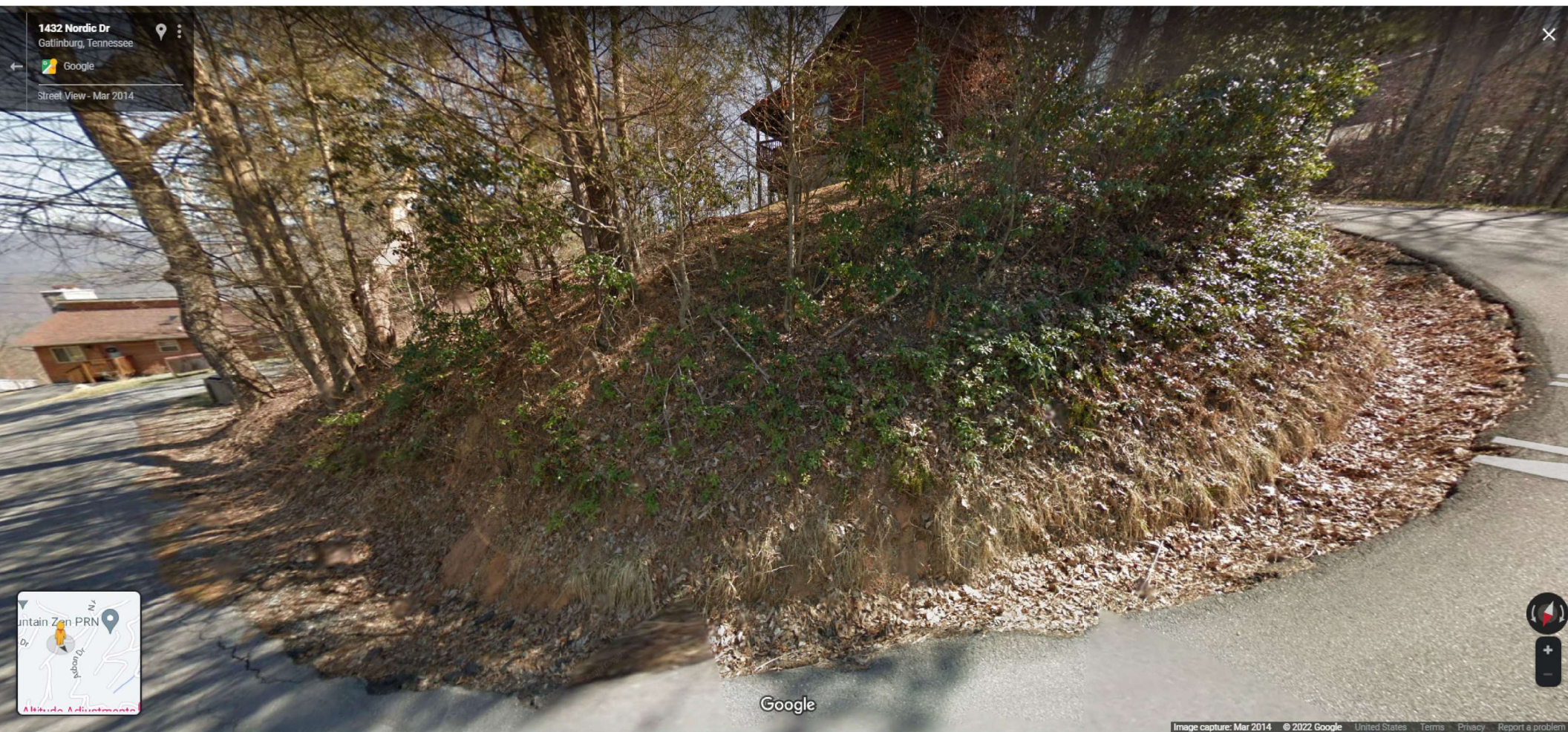
VIEW OF SWITCHBACK FROM OUTER RADIUS
