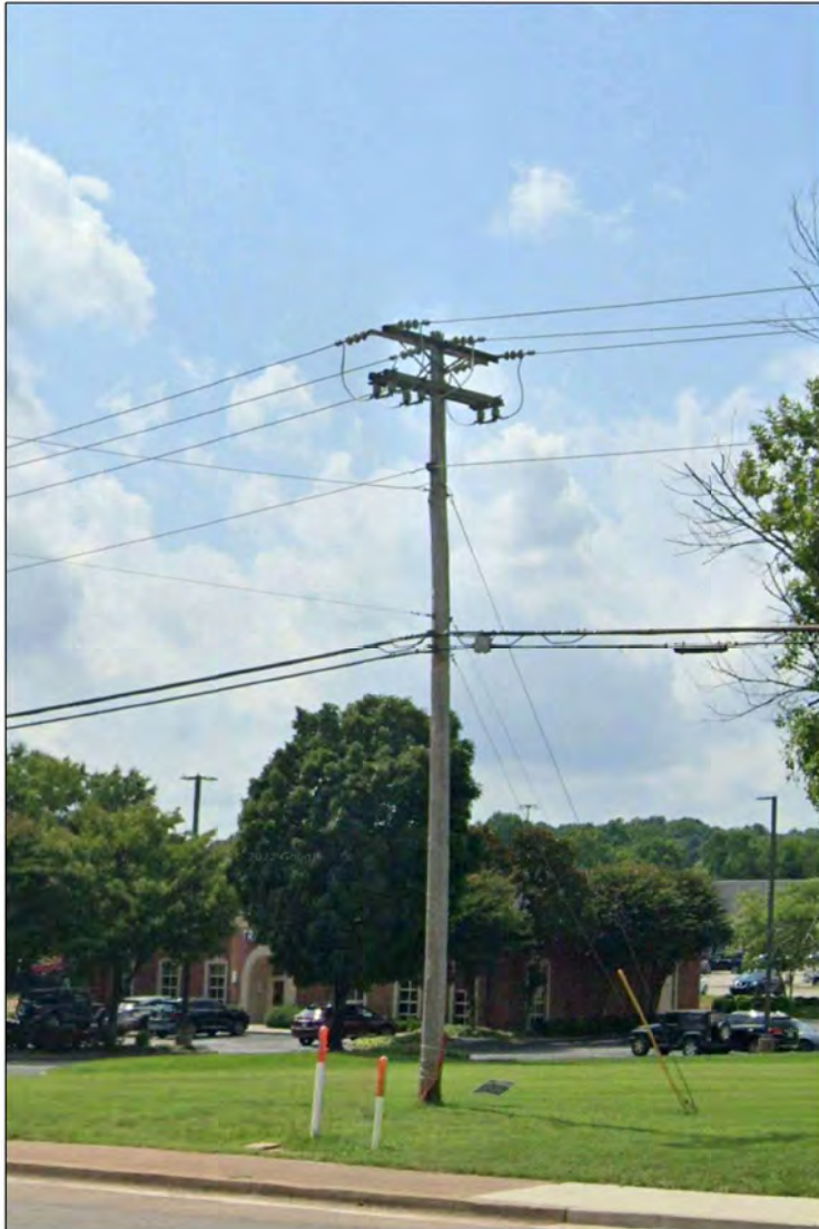
1 CURRENT VIEW (FROM EAST LOOKING WEST)
