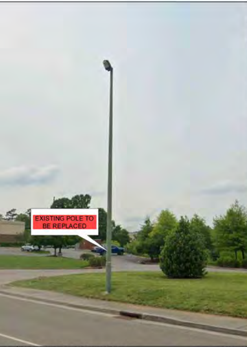
1 | POLE LOCATION PHOTO
