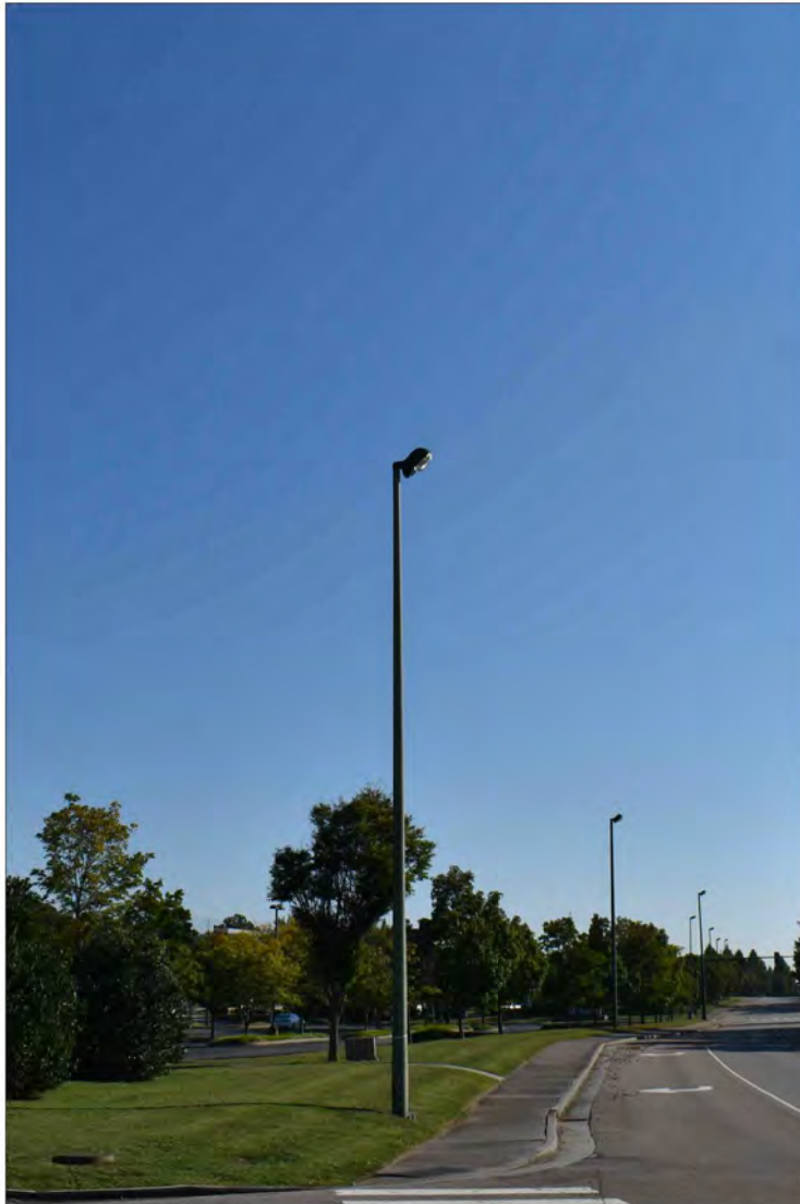
1 CURRENT VIEW (FROM WEST LOOKING EAST)
