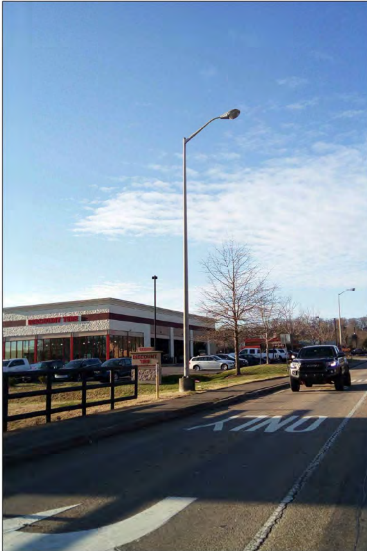
1 CURRENT VIEW (FROM SOUTHEAST LOOKING NORTHWEST)
