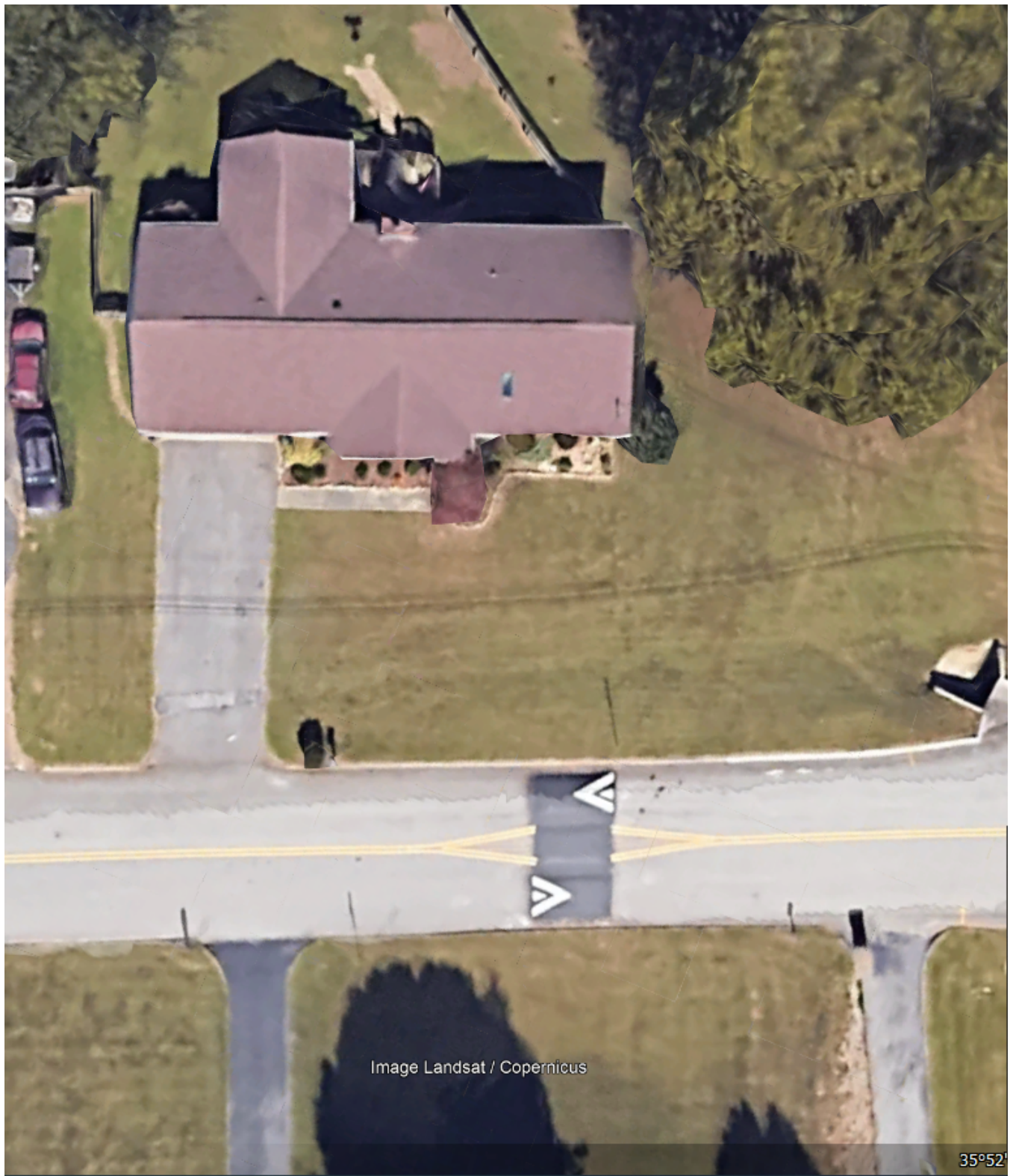
Midhurst Road Speed Cushions installed in 2022
