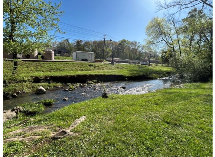
Project Site April 2025
