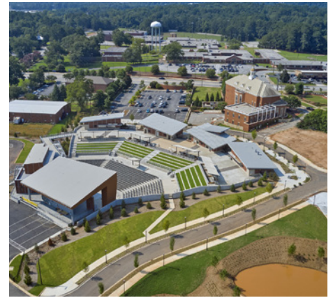
City of Stockbridge Amphitheater and Park - Atlanta Regional Commission Livable Center Regional Excellence Award
