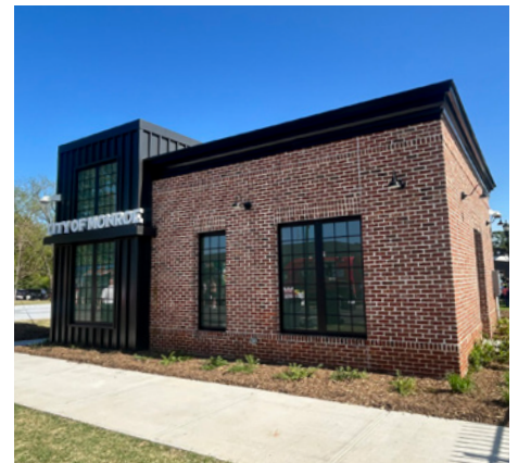
City of Monroe Town Green (includes an Amphitheater and Restrooms)
