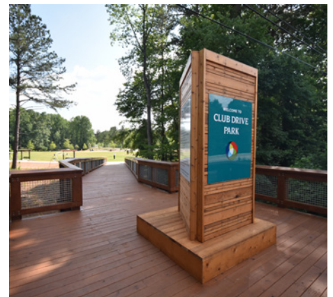
Gwinnett County Club Drive Park Phase II Boardwalks and Connection to Sweetwater Creek Greenway
