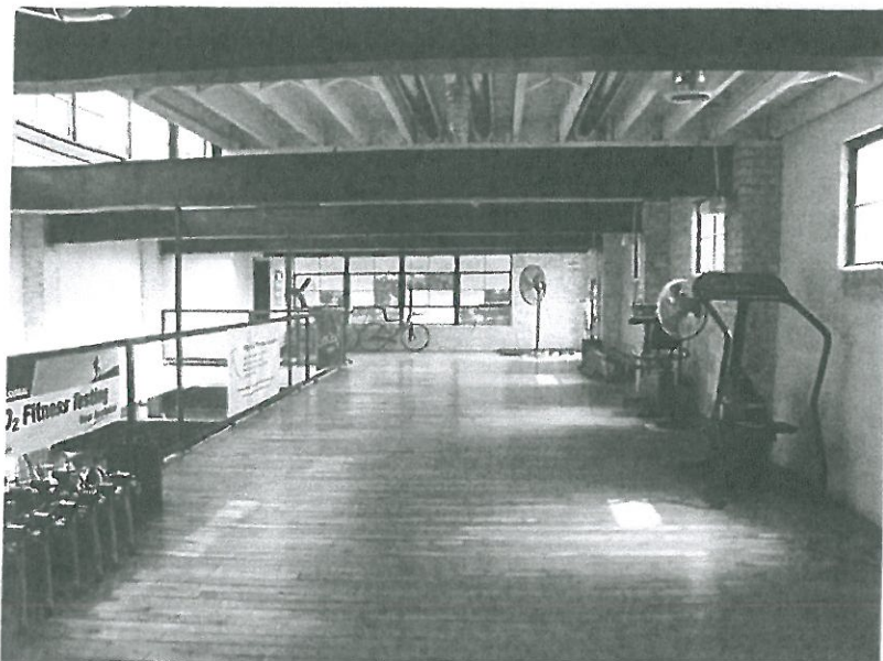
Second level space used for classes. Remodelers discovered this previously unknown space.
