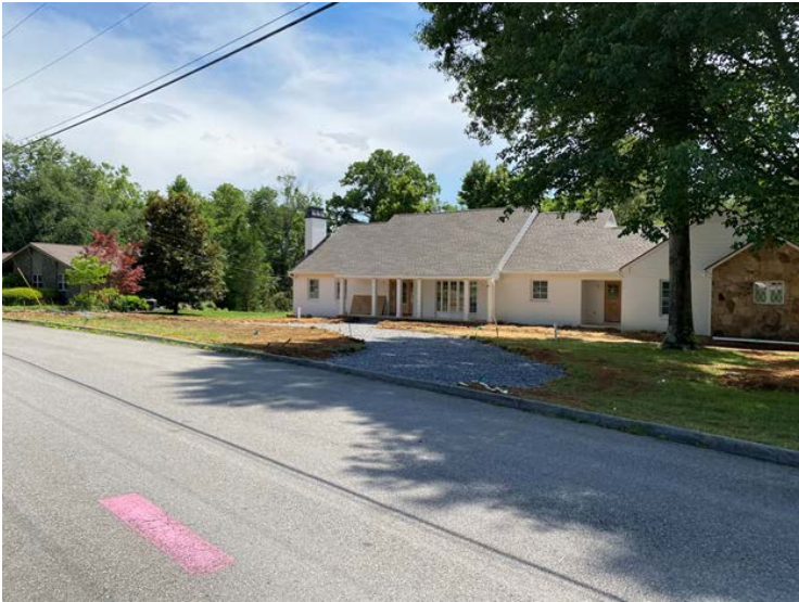
Monticello Drive right view of circular drive
