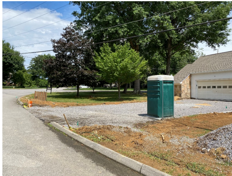
Weathervane Drive approach to Monticello Drive right turn
