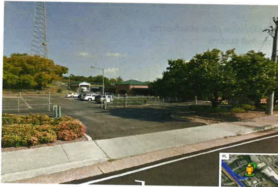
Photo of Emergency Operations Center entrance- 605 Bernard Ave. Knoxville TN
